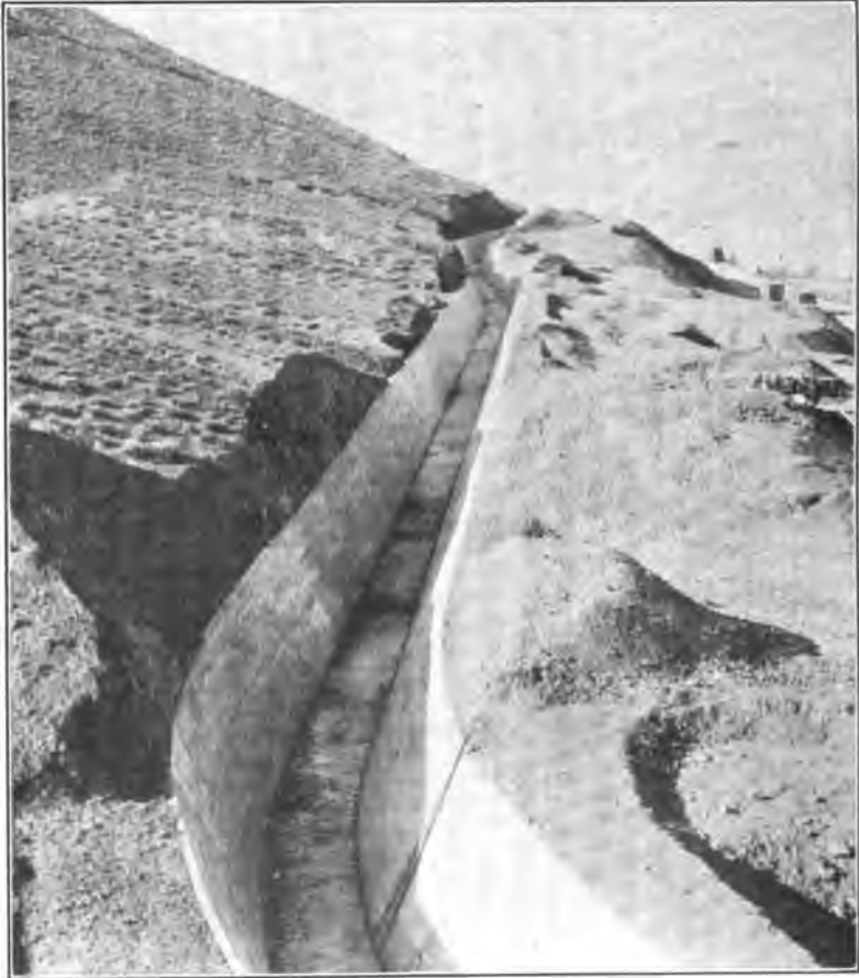
FIG. 81.—Concrete Lining, Truckee-Carson Canal, Nevada.
